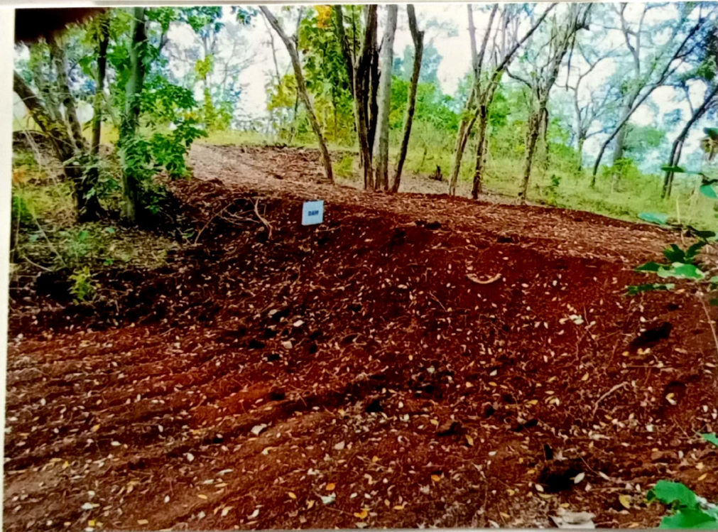
DAM at. College Premises.
