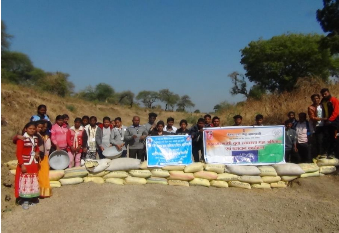
Check Dam Construction Across a River
